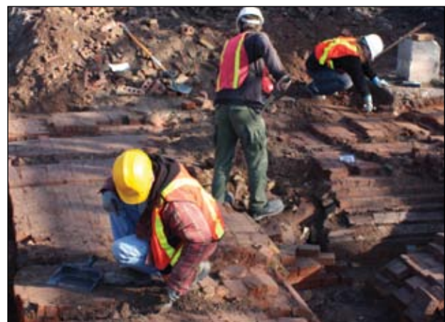
Construction at the Brick Works.
